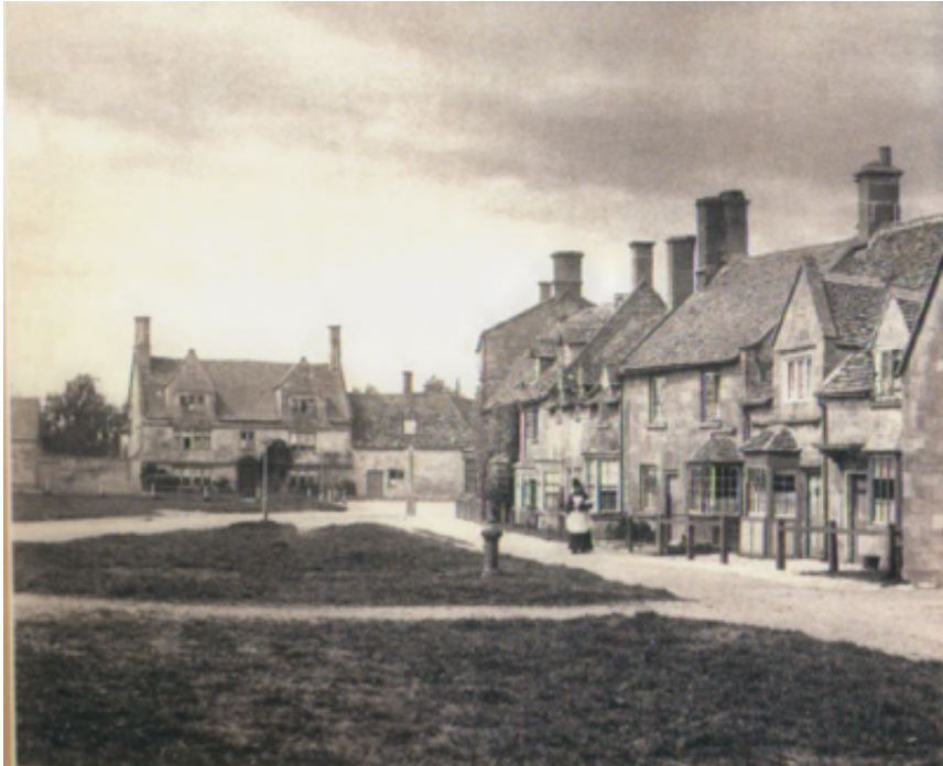
View of Farnham House from the Green, Broadway, 1896 (Houghton, Broadway Pictorial)
